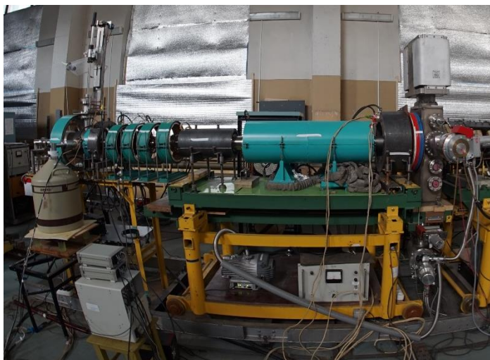
Installation of the Positron Injector DLNP JINR
